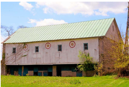
Bieber Barn on Stratford Road
