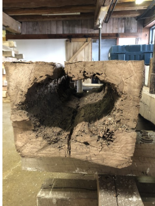
Rotted beams removed
