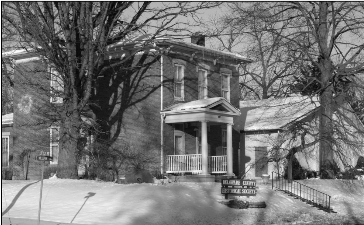
The Cryder Historical Center includes the Nash House, left, and the library/annex building
