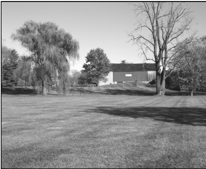
The Stone-End Barn at the Meeker Homestead
